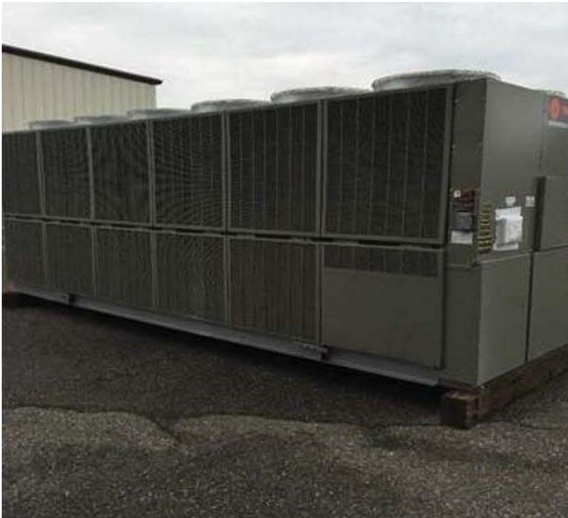
Example of a 200-ton heat capacity chiller
