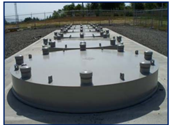
Figure 2: Holtec’s Underground Dry Storage System at Humboldt Bay
