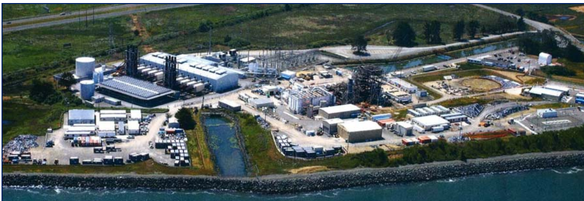
Figure 3: Humboldt Bay hosts World’s First Underground Storage Facility by Holtec (2007)
