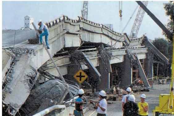
**Fig. 3. Cypress Street Viaduct Before and After Collapse**
