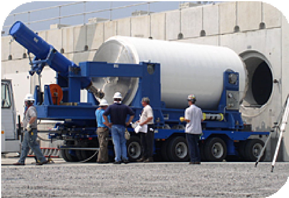
Fig. 3. NUHOMS canister fits inside a concrete overpack.
