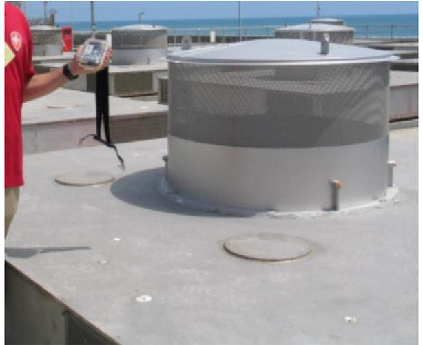
*Large air vents in Holtec lids allow corrosive marine environment to corrode canisters and start the cracking process.*
