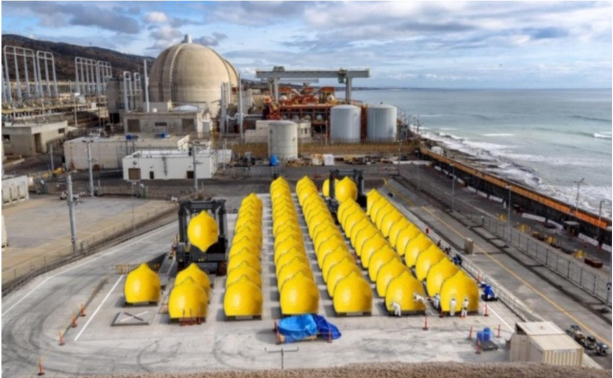
The Nuclear Regulatory Commission (NRC) admits in their November 28, 2018 NRC Inspection Report and Notice of Violation, ML18332A357 (page 8 and 9) every Holtec canister downloaded into the storage holes is damaged due to inadequate clearance between the canister and the divider shell in the storage hole (vault). The NRC states canister walls are already “worn”. This results in cracks. Once cracks start, they continue to grow through the wall.
